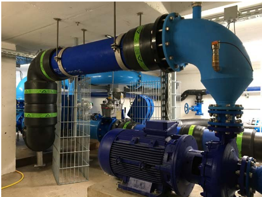
Figure 8: Condition at Surge tank after Installation
