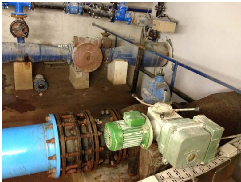
Figure 6: Before Installation condition at Surge tank
